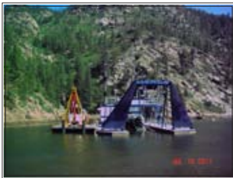
Strontia Springs dredging rig
